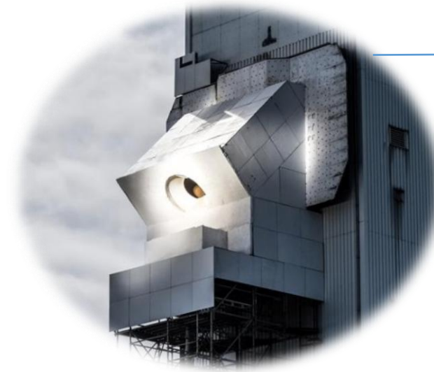
DLR's 1000° C direct absorption particle receiver (DLR)
